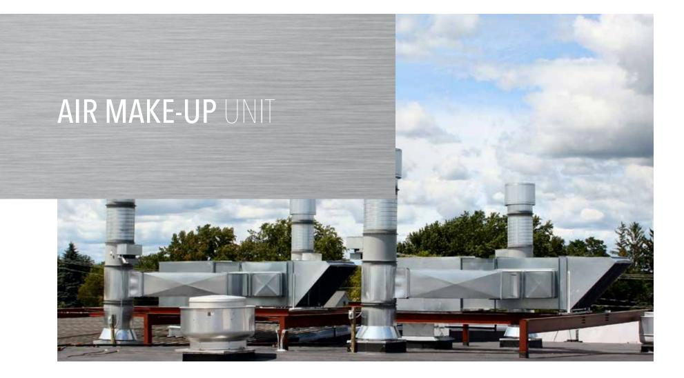
GFS' direct gas-fired air make-up units (AMU) provide an economical source of replacement air. By continually replacing contaminated booth air with fresh, heated outdoor air, AMUs maintain a constant air temperature regardless of the air temperature outside your building. This allows for balanced building pressure and proper comfort levels.
